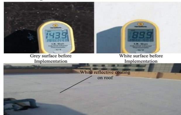
Figure 3 Heat Load Reduction Through Reflective Coating
