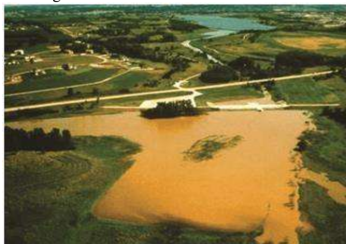
Figure 3 Muddy Water in Tank
